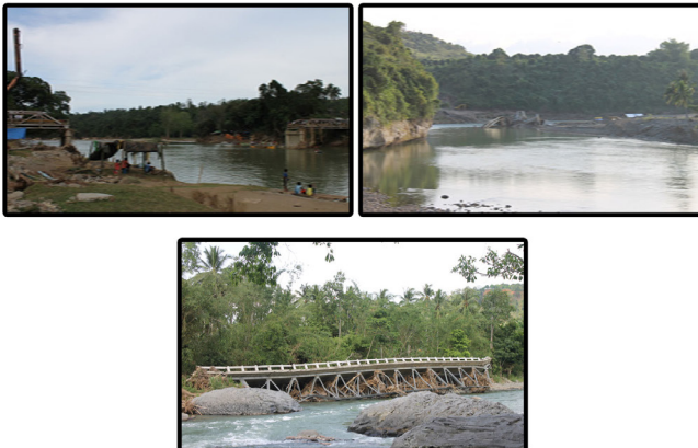
Plate 1. Station 1: Dansolihon - Uguiaban Bridge.
