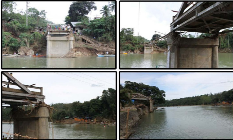
Plate 2. Station 2: Lumbia - Cabula Bridge
