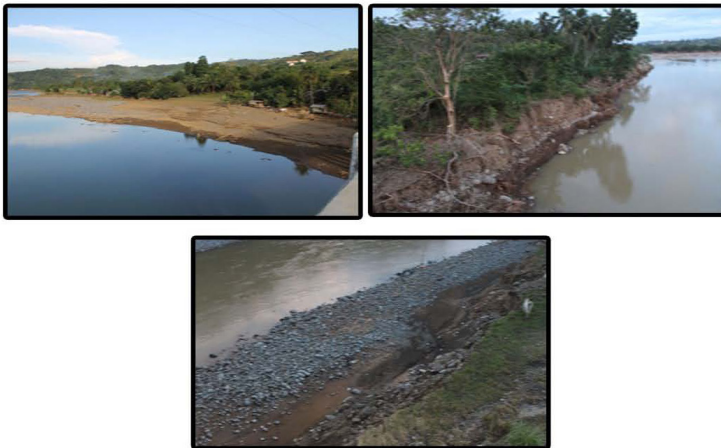
Plate 3. Station 3: Taguanao - Taguanao Bridge
