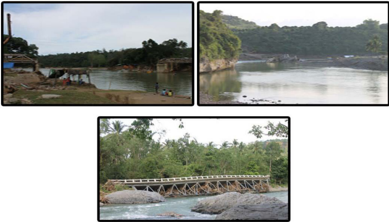
Plate 1. Station 1: Dansolihon - Uguiaban Bridge
